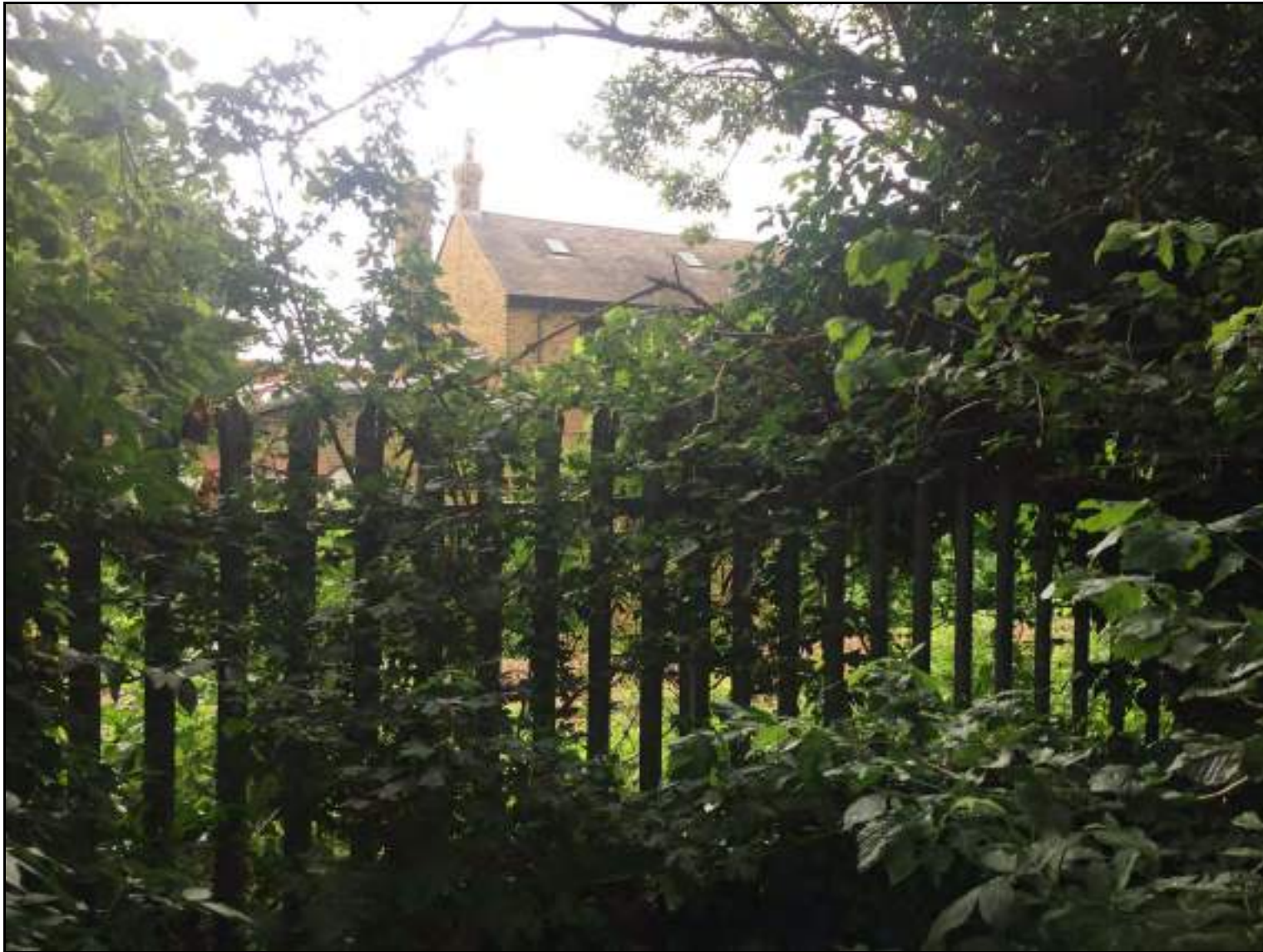
Fig. 23 Railing at top of embankment (2021)
