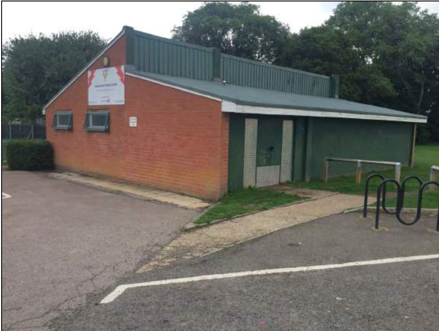
Fig. 16 The football pavilion (2021)
